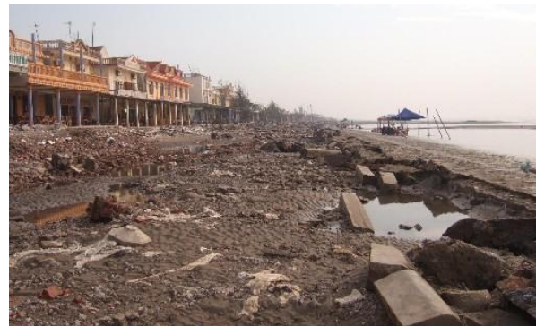
Figure 3: Hai Hau coastal resort in Red River Delta was damaged by erosion
