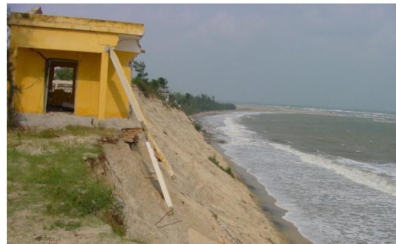
Figure 4: Erosion in sandy coast of Hai Duong Village Thua Thien Hue Province, Vietnam Centre
